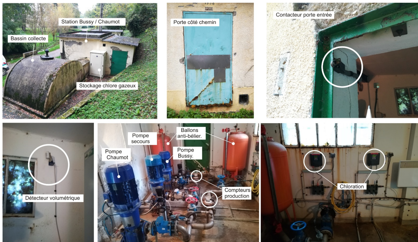
Figure 5 : station de pompage de Bussy-le-Repos / Chaumont.
